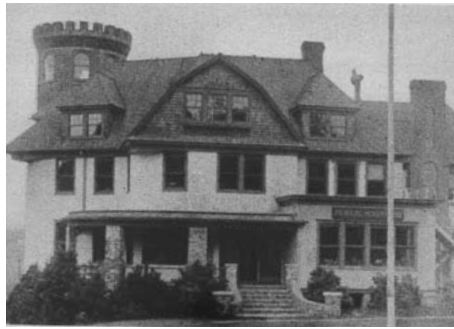
The soon-to-be demolished Van Vliet house, 1930.
